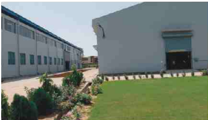
CoilCo - Manufacturing & Assembly-section plant in India Plant-I in New Delhi & Plant-II in Gurgaon - Haryana
